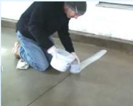
Most concrete floors have cracks and pits from years of wear and salt erosion. We fill them with a thick coat of epoxy to eliminated these unsightly imperfections.
