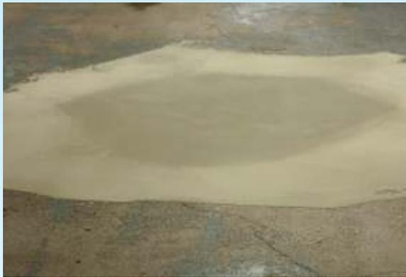
Some floors may have major surface damage spots that require repair and leveling. We use a high tech cementitious composite epoxy, resulting in a very strong repair, stronger than the original concrete.
